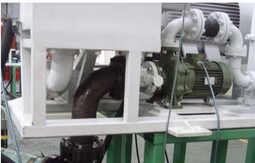
NR. 1 IR CHINA PUMPS ARE INTEGRATED INTO MACHINERY FOR CERAMIC PROCESSING
